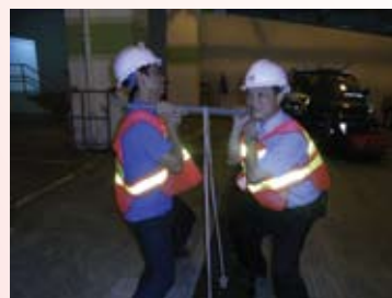
○ 每個排骨渠蓋可重達20公斤，加上渠蓋之間緊密連接，令員工拉起渠蓋時感到十分困難，甚致容易引致受傷。 Surface channel covers may reach 20kgs each and they are tightly trapped. It is therefore hard for the staff to lift up these heavy surface channel covers while they are easily prone to injuries.
