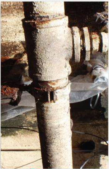
塗上防銹蝕修護物料後的立管 Riser applied with a rust-preventive coating
